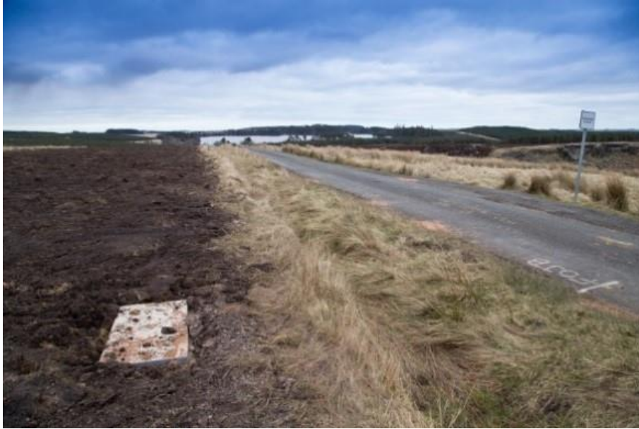
Plate 2 Example below ground link box following reinstatement (Source: Rey Wind Farm, Vattenfall Wind Power Ltd.)
